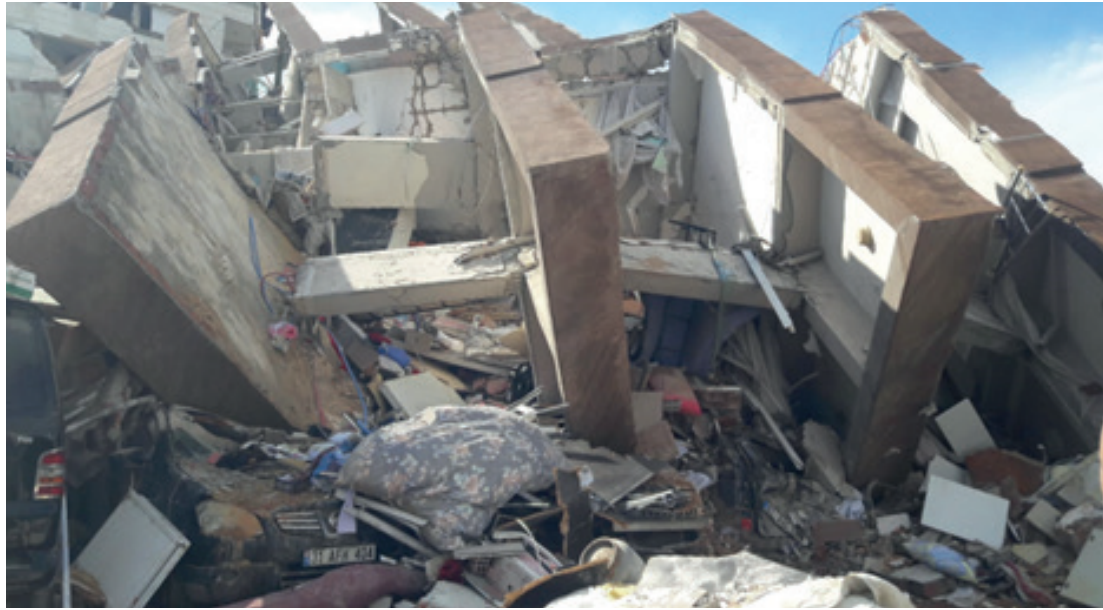
Fuat Koku, after the earthquake
