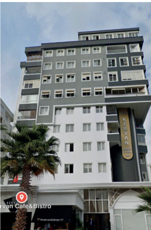
Ezgi Apartment, before the earthquake
