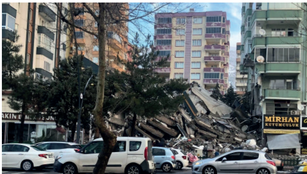
Fazilet Block A, after the earthquake
