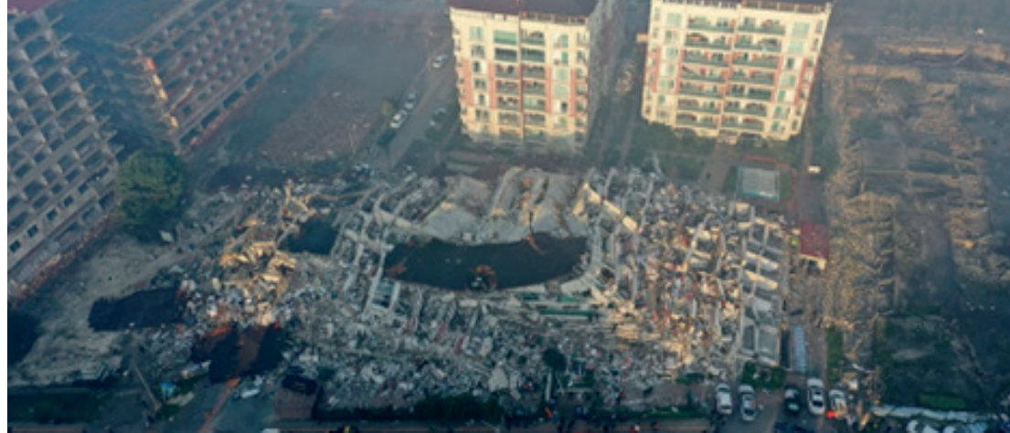
Rende Block A and Block B after the earthquake (Sözcü)
