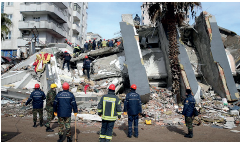
Ezgi Apartment, after the earthquake (TRT HABER)
